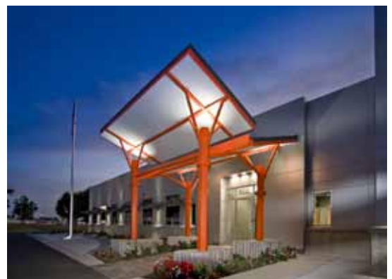
Circa 2011 - Old Missouri Road Plant - Springdale, AR
